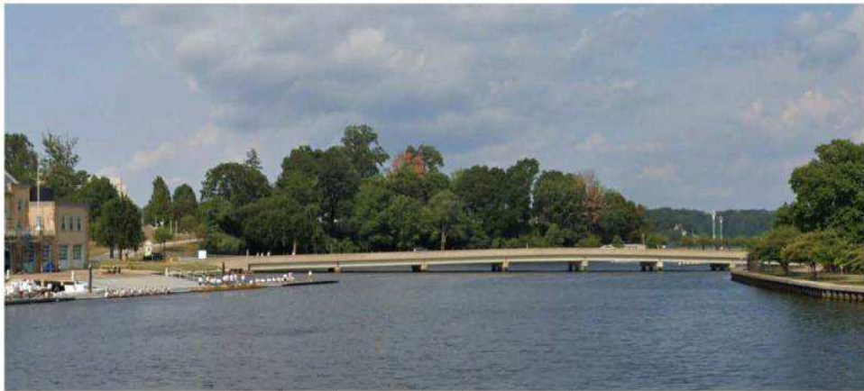
Decatur Avenue Bridge, east view
