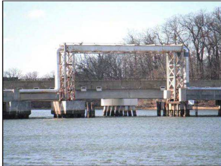
King George Street Bridge and Utility Bridge, west view
