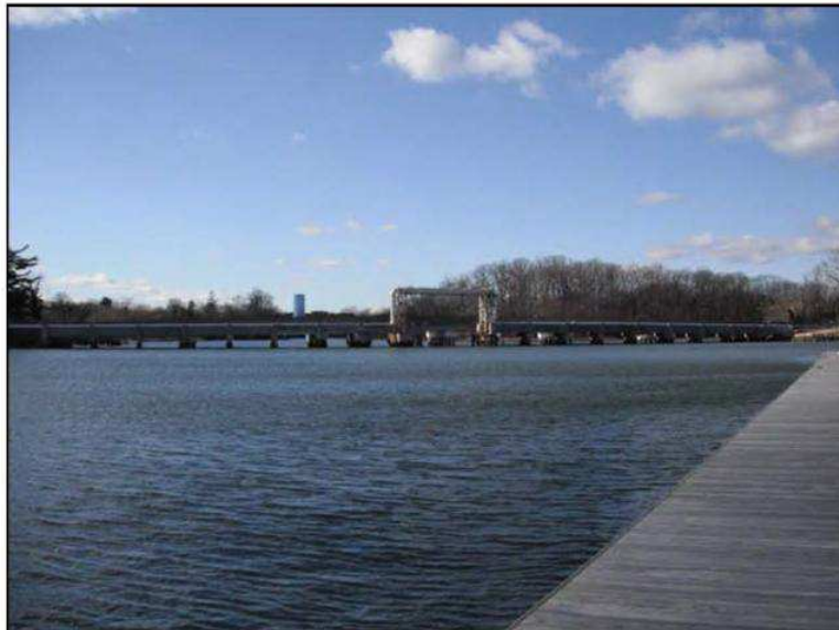
King George Street Bridge and Utility Bridge, looking west
